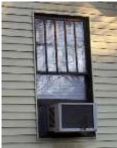
Window mounted AC should be mounted on side or rear of building.
